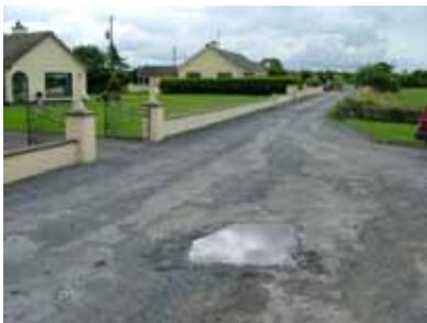
**Photo 16:** The occasional pothole is evident on road edges and road junctions. Otherwise roads through the village are in very good condition.
